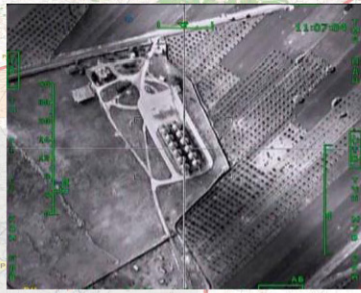
Oil storage facility near Al Thawrah settlement
